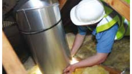
Once in place, seal ALL the remaining seams and joins with the aluminium tape provided.
