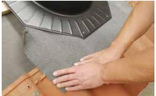
Ensure the flashing is clean and dry, then peel away the protective backing film from the Solafoam weather strip and apply it to the roof flashing as shown.
