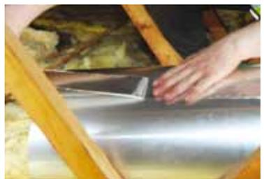
Use the shiny side of the tape's backing paper to rub over the aluminium tape to produce a smooth, well-bonded surface on all joins.
