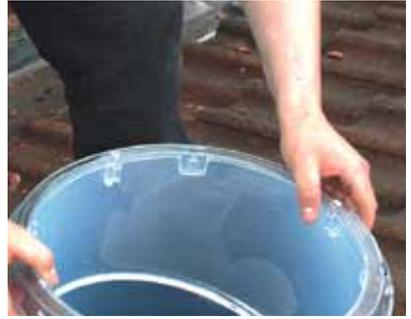
Screw the dome ring to the up-stand through the pre-drilled holes using the screws provided and remove the protective film from the inside of the top tube assembly.
