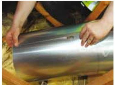
Assemble the required length of extension tubes to join the top tube to the ceiling tube, ensuring a minimum of 50mm overlap between each join. Use small pieces of tape to hold the tubes together. Check the assembled tube length is correct and fits into the top and ceiling tubes. All extension tube joins can now be fully taped.
