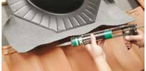
Apply hand-pressure to form the Solaflex flashing sheet to the profile of the tiles below.
