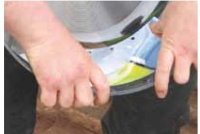
Keeping the LightTracker™ dome reflector on the north side of the dome facing south, align the four locking tabs on the dome base with the snaps on the dome ring. Press down firmly until the dome locks into place. Ensure the tabs are fully engaged.
