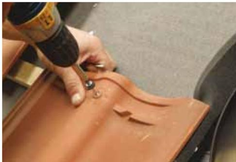
Cut the remaining tiles to fit around the top of the flashing, ensuring there is a minimum gap of 40mm between the tiles and the up-stand to allow the Solatube® roof dome to be fitted (see dome and top tube assembly installation section for more details on page 8). Ensure all the replaced tiles are firmly in position and watertight.
