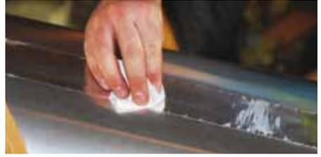
On the uppermost extension tube, wrap the self-adhesive expansion joint seal twice around the outer diameter of the tube, approximately 25mm from the top. If no extension tubes are used, the expansion joint seal is applied to the ceiling tube assembly.
